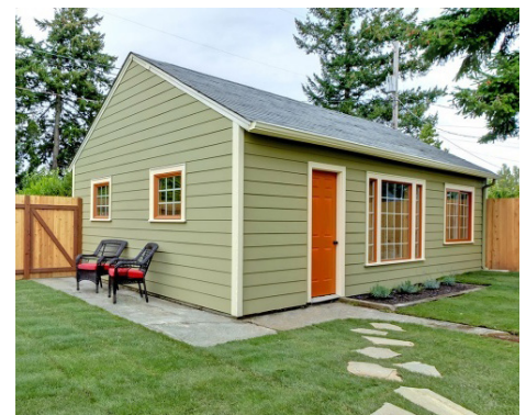
Accessory Dwelling Units like this one are often accessed from the alley. Source: Neighborhoods.com
