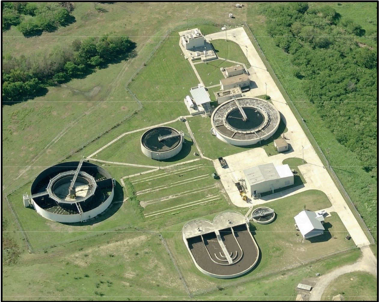
Figure 4. “Bird’s Eye” View of WWTP Property
