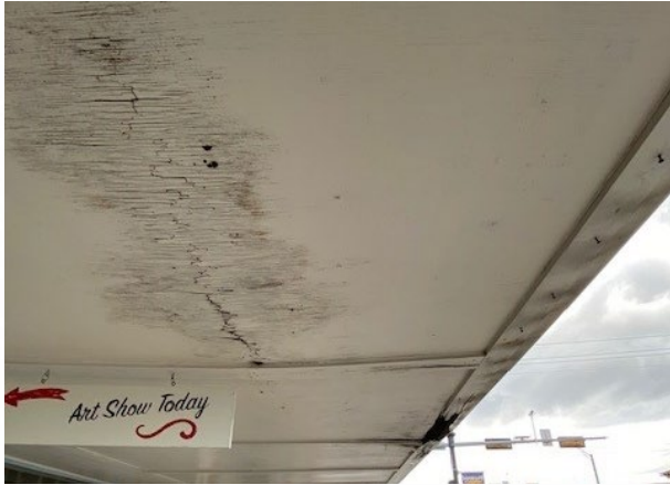
Façade Improvement Grant 50/50 Match up to $5,000
