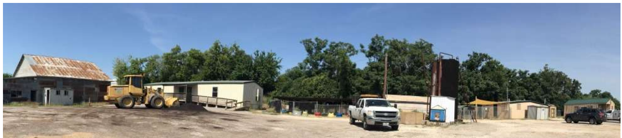
From left to right: Storage Barn, Portable Storage Building (from Taylor ISD), Outdoor Dog Kennels, Laundry/Cat Room, Indoor Kennels, Food Storage Shed and Shelter Office.
