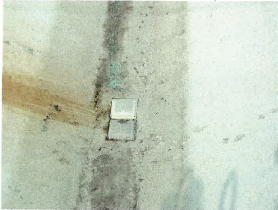
Photo of Main Drain grate covers
