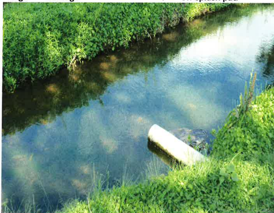
Image of discharge pipe from swimming pool backwash
