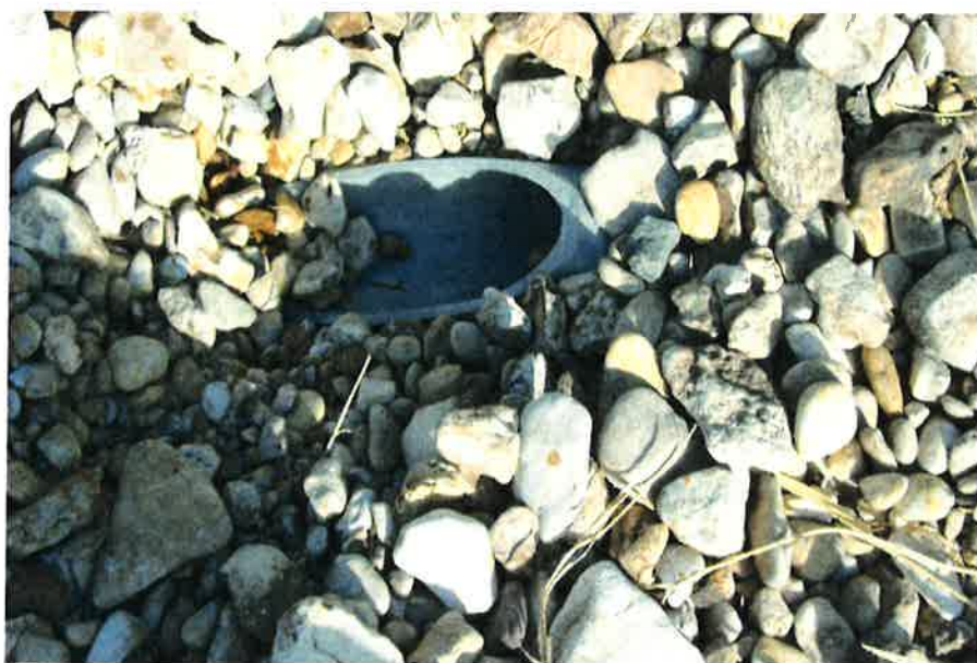
Image of discharge of backwash flow from new splash pad
