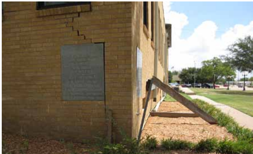
Wood supports on the south wall
