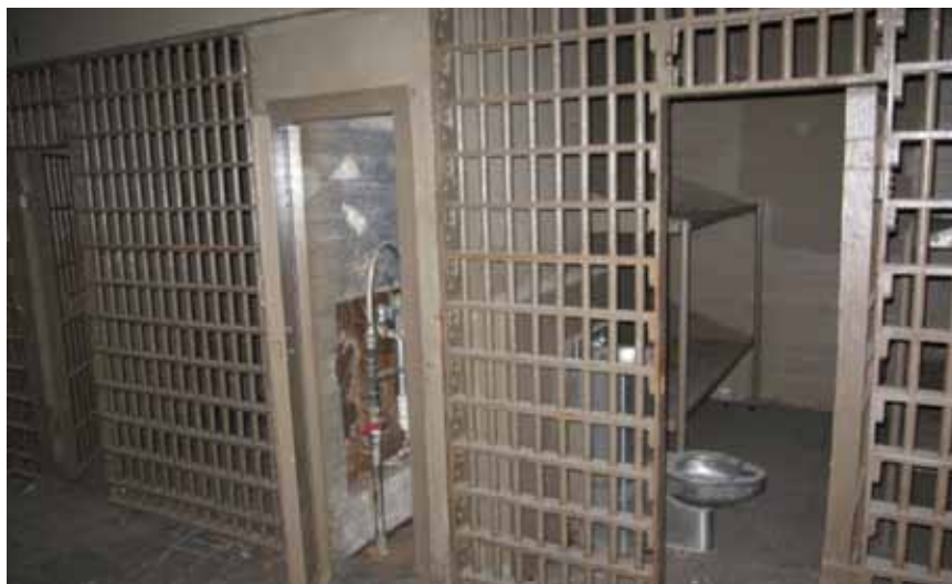
Jail cells in south portion of basement
