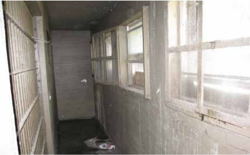
South windows at the basement jail area
