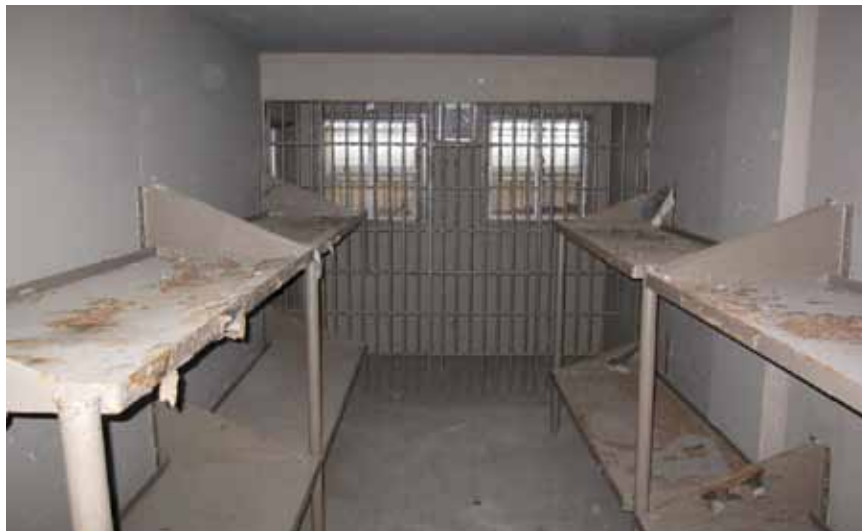
Jail cells showing bunks at north portion of basement
