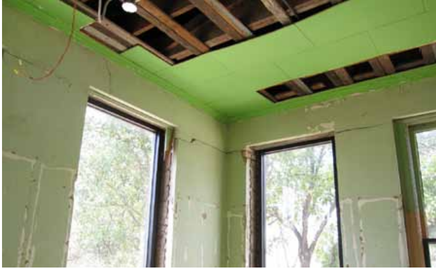
Windows and ceiling at former Police area
