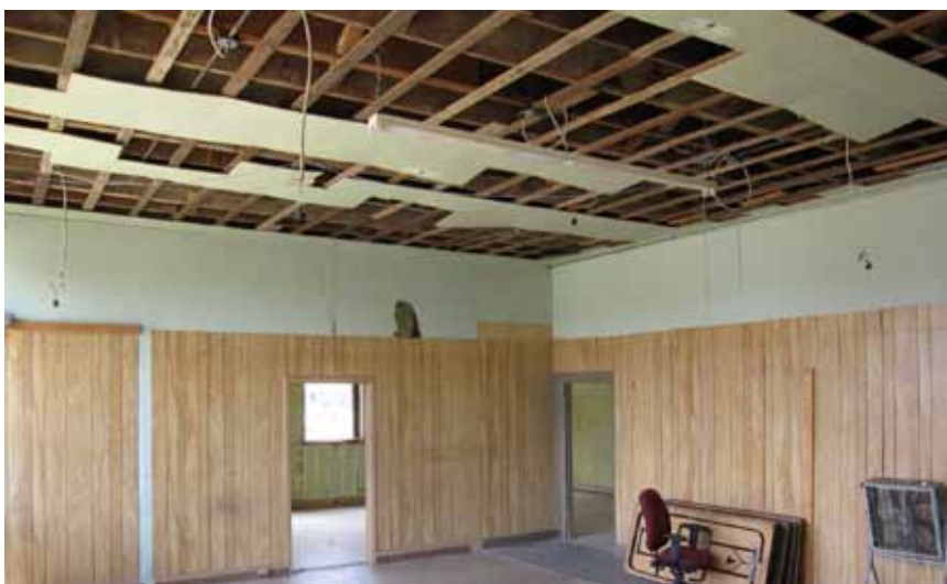
Main office of former Police area
