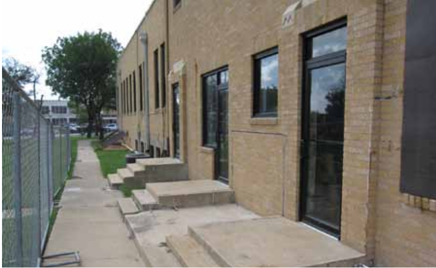
South wall of former Fire Station
