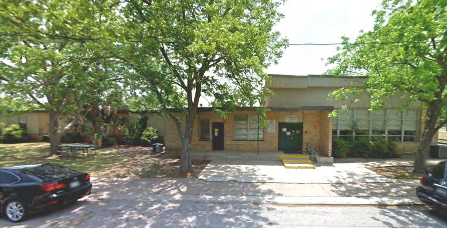
Figure 9 – “Band Hall” Annex Building – Site C
