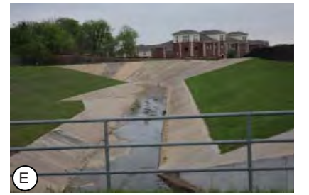
(E) Drainage ditch at the back of new homes
