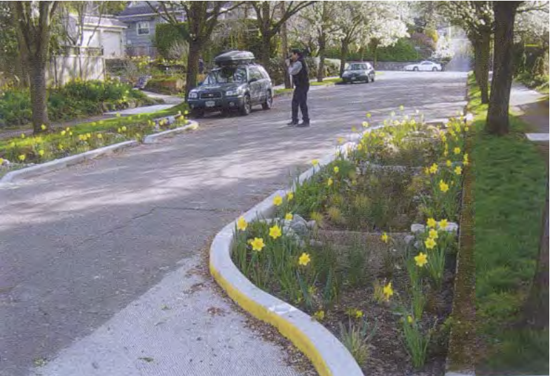
Bioswales in residential bulb-outs become an extension of the front yard amenity.
