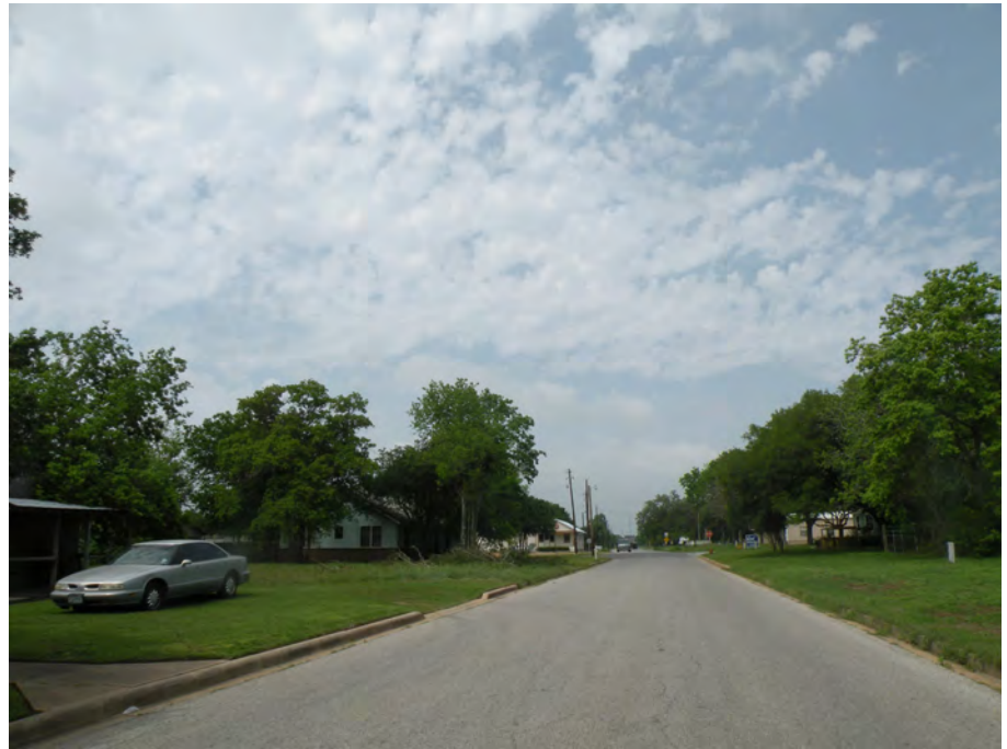
Streets lack sidewalk connectivity.
