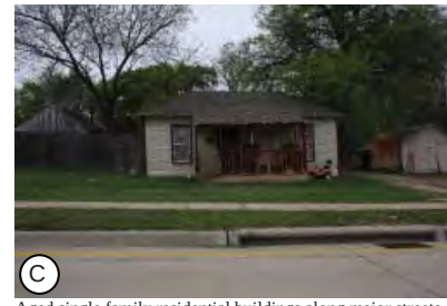
(C) Aged single family residential buildings along major streets
