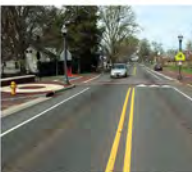
Traffic Calming and Lighting
