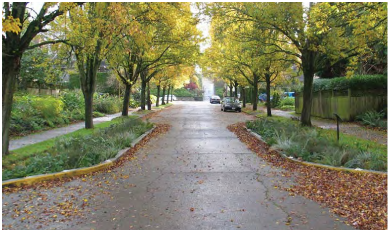
Bulb-outs are designed with rain gardens and bioswales to filter contaminants from the street.
