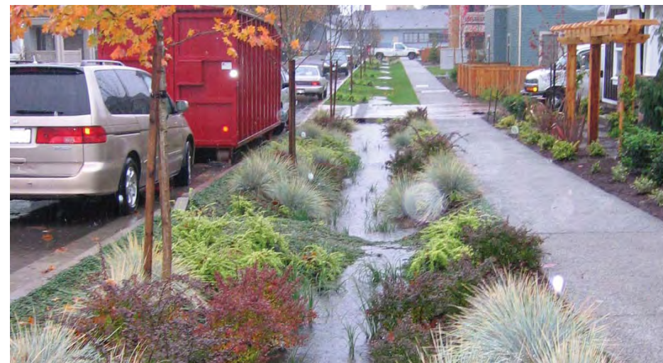
Nature strips are transformed into bioswales.
