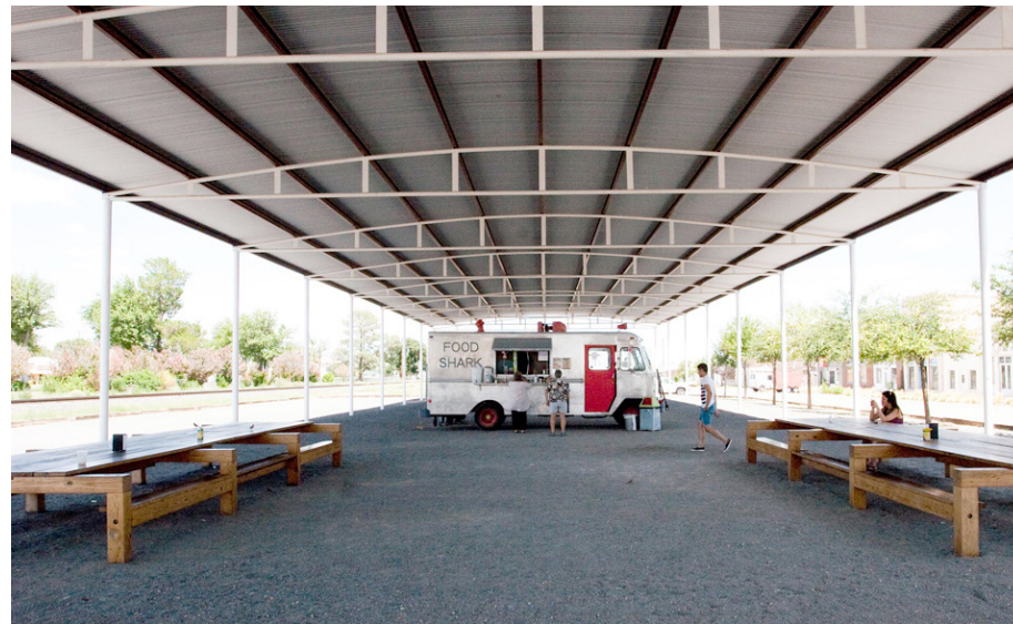
Industrial Shade Structure / Flexible Space
