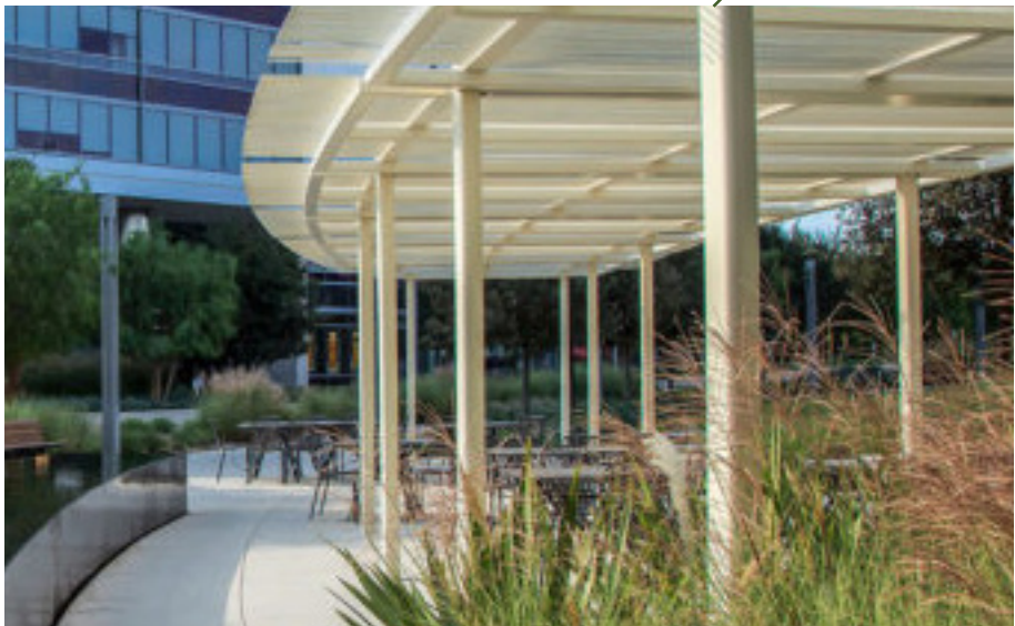
Steel Shade Structure
