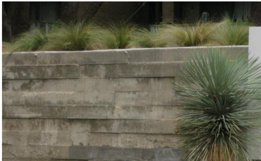
Bowl Retaining Wall
