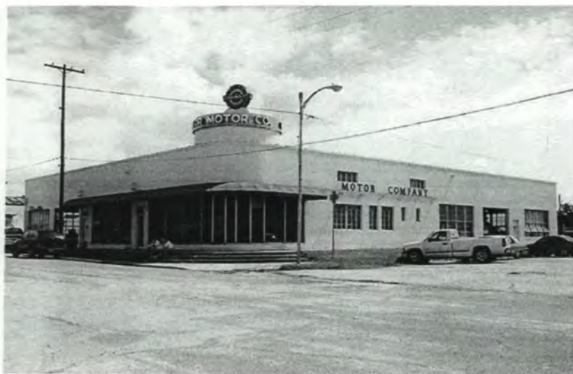
Taylor Motor Company (1930-31) 200 Porter Street Property #32 Streamline Moderne Contributing Photo #10
