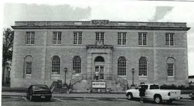
United States Post Office (1929-30) 202 West Fourth Street Property #88 Central Block with Wings / Classical Revival Contributing Photo #11
