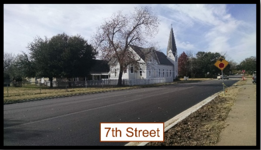
2019 Street Maintenance Project
