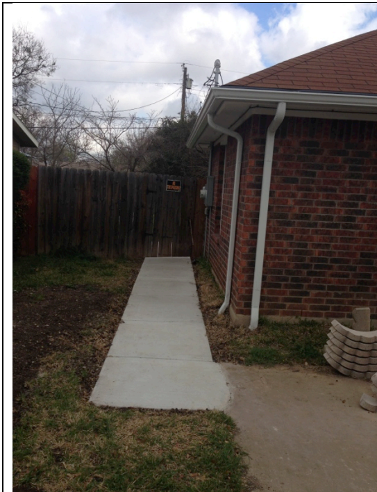
View of new walkway through gate to back yard, along the side of the home and connection to back of driveway.
