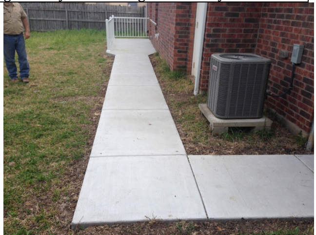
View of new walkway as it turns to side of home through gate.
