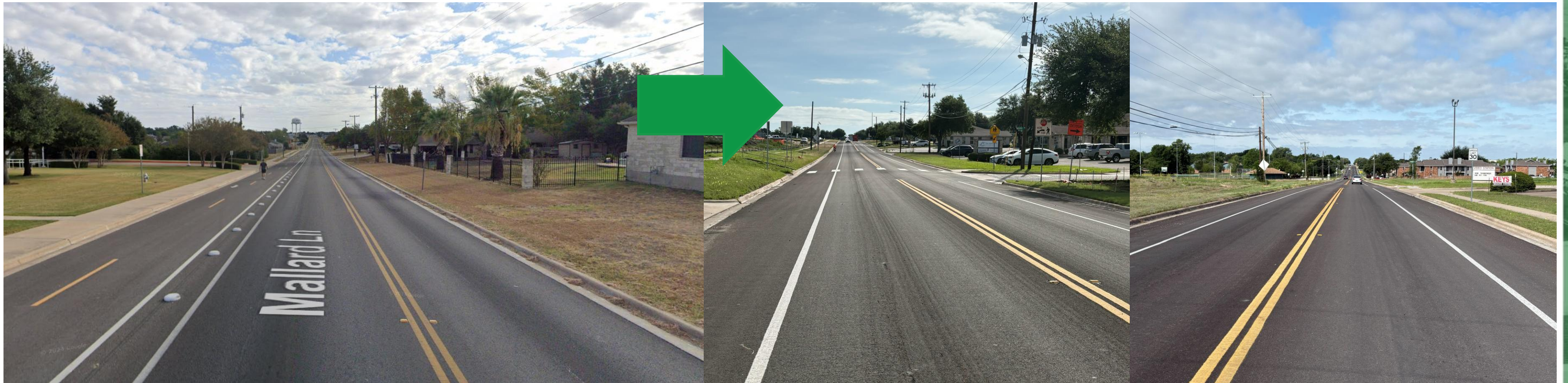
Previous pavement markings and concrete buttons, looking east from North Dr
