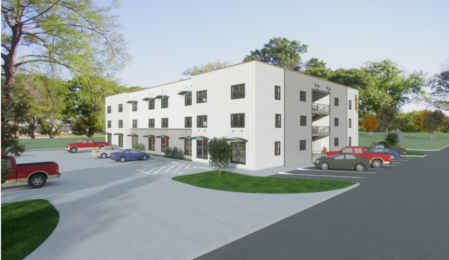
W 3 rd St looking south-west
