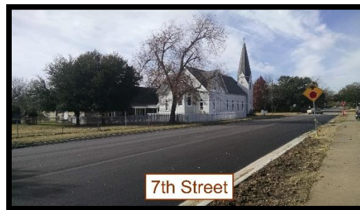
2019 Street Maintenance Project
