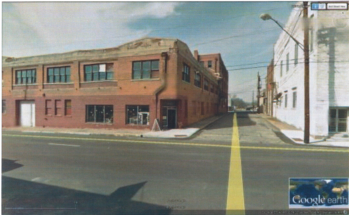
Rogers – Wade Building – 204 Grand Avenue – Paris, Texas
