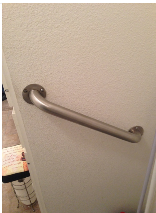
Tightened grab bar to the side of toilet.
