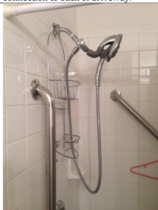
New shower wand. Note tightened grab bars.
