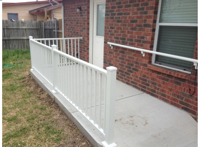
Alternate view of rear wheelchair ramp gradually descending to walkway.
