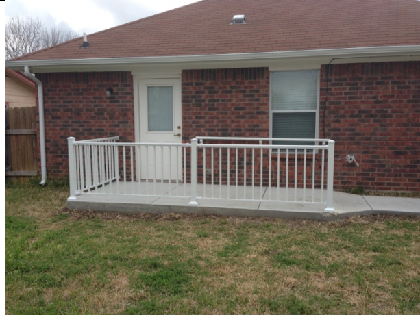
New rear patio, concrete wheelchair ramp and metal guardrails.
