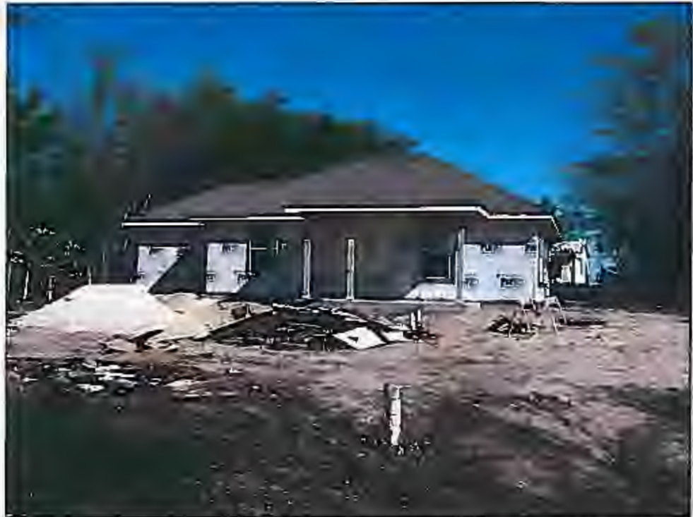
HOME HRA – Construction of a new home administered by LCMS
