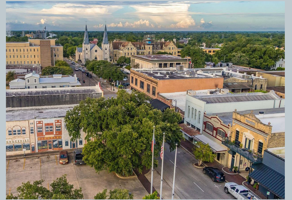
Victoria uses grants, tax incentives, and financing programs to boost downtown revitalization and infill development.
