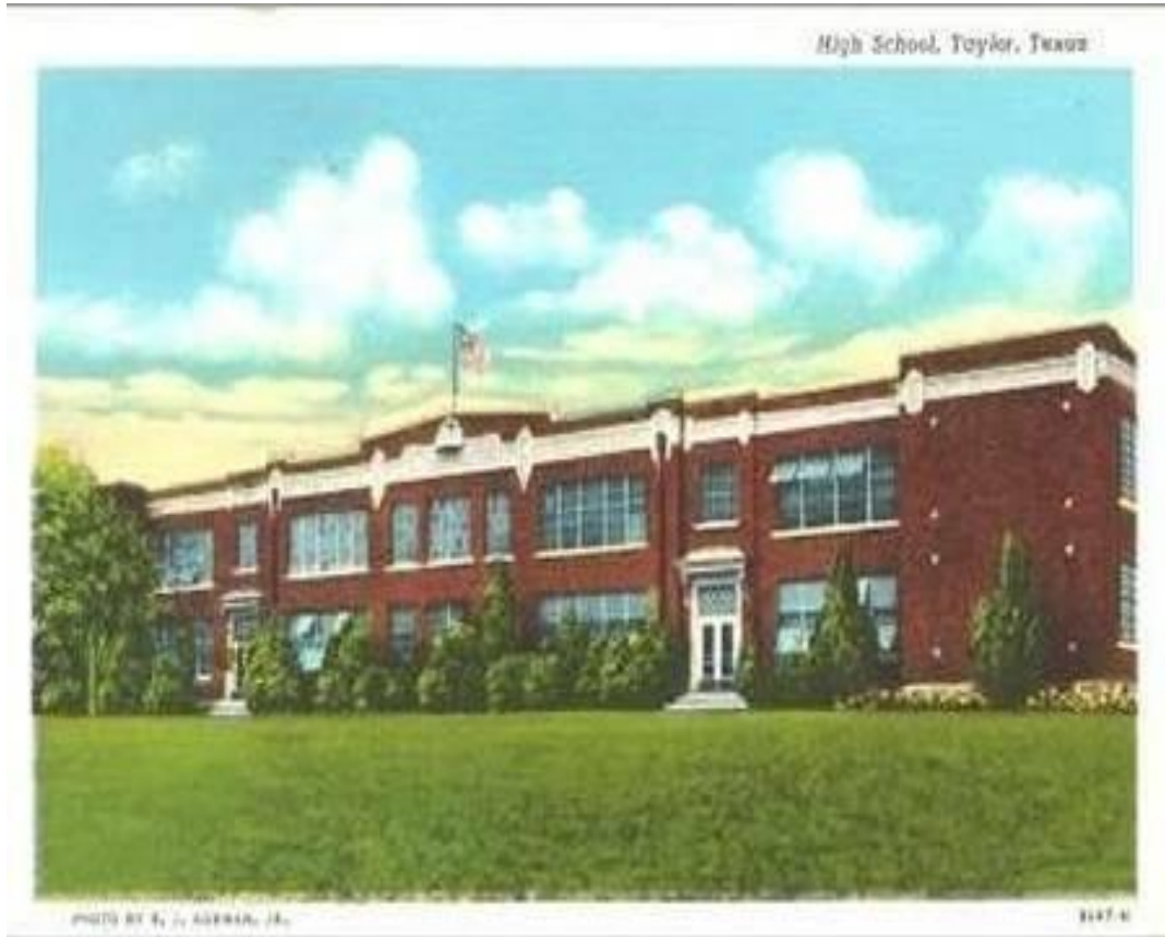
Figure 7 – Campus Main Building
