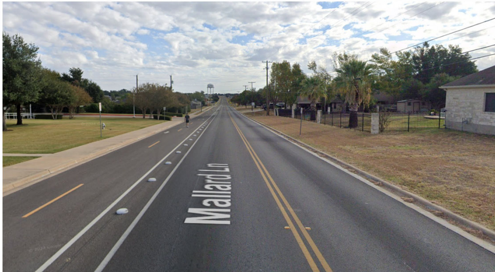
Existing pavement markings, looking east from North Dr
