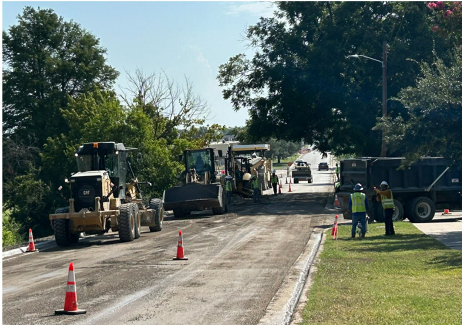
(Lake Dr – Pavement reclamation work)
