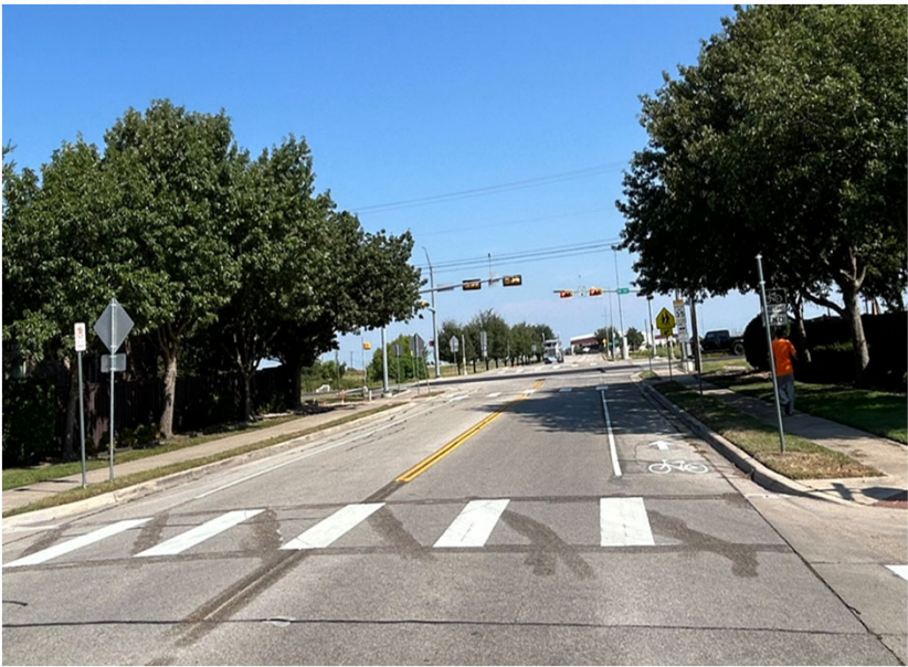
Water Blast Removal – Bill Pickett Trl.
