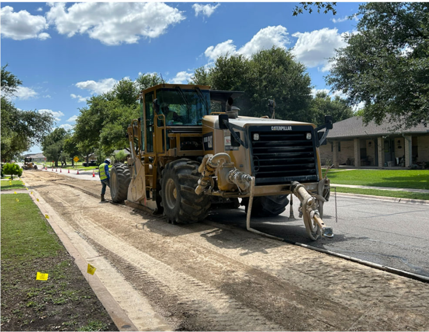
(TH Johnson – Pavement reclamation)
