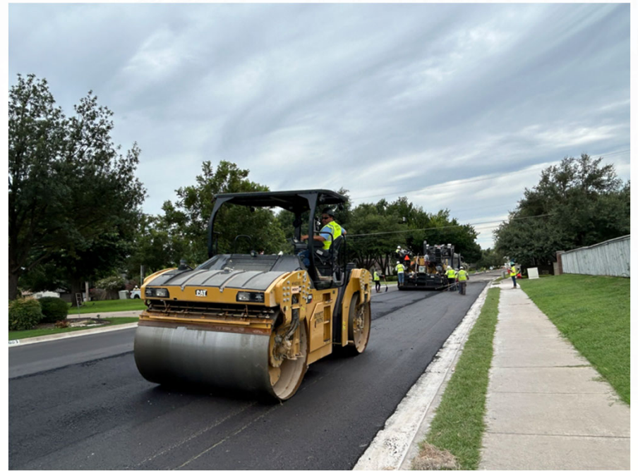
(TH Johnson – Hot mix asphalt paving)
