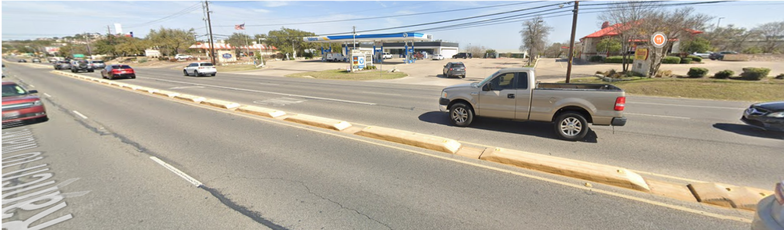
Example Implementation: RM 620 in Lakeway, Texas
