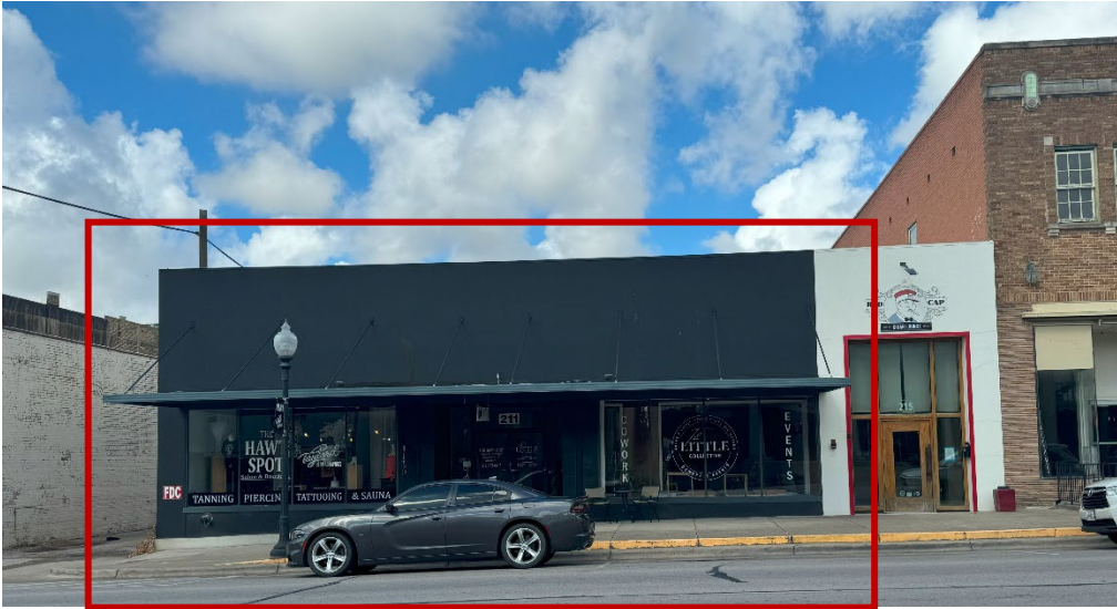
Current Front Façade.
