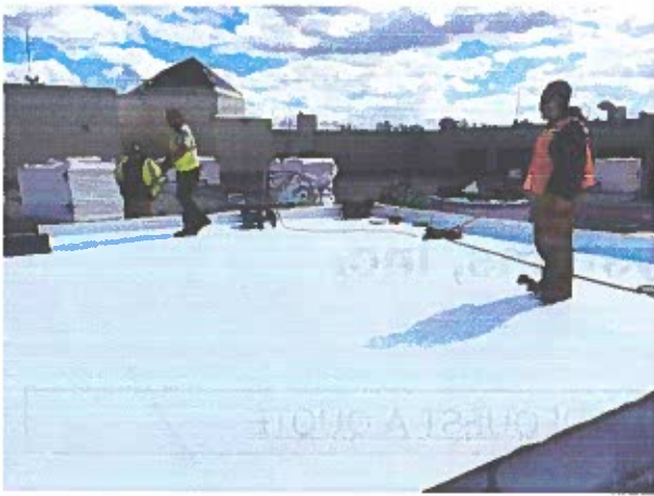
In-progress photo of a TPO roof installation
