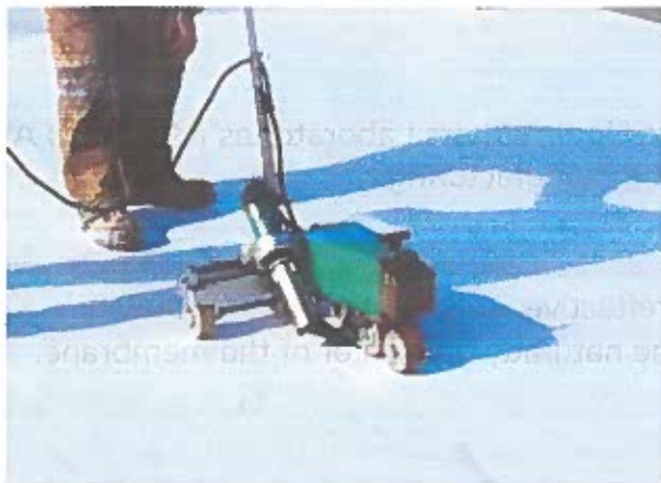
Seams of TPO roof being heat-welded together
