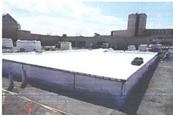
Finished TPO roof section
