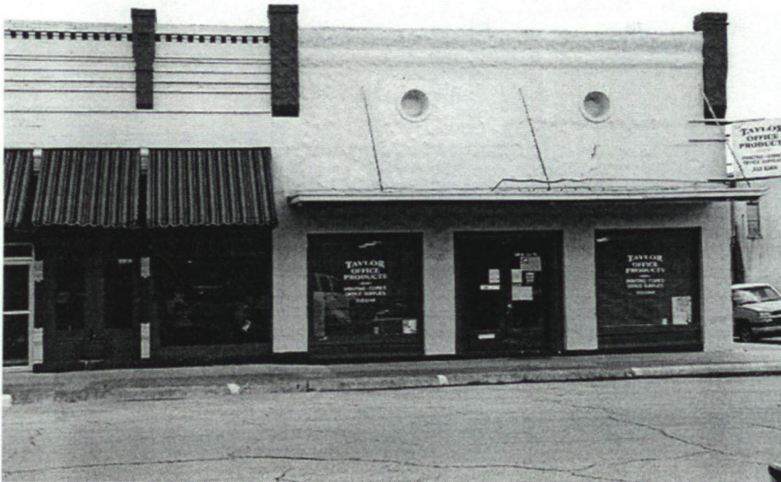
Taylor Office Products Building / Richter Furniture (ca 1904) 119 West Third Street Property #46 One-part commercial Non-contributing Photo #14 and Photo #15
