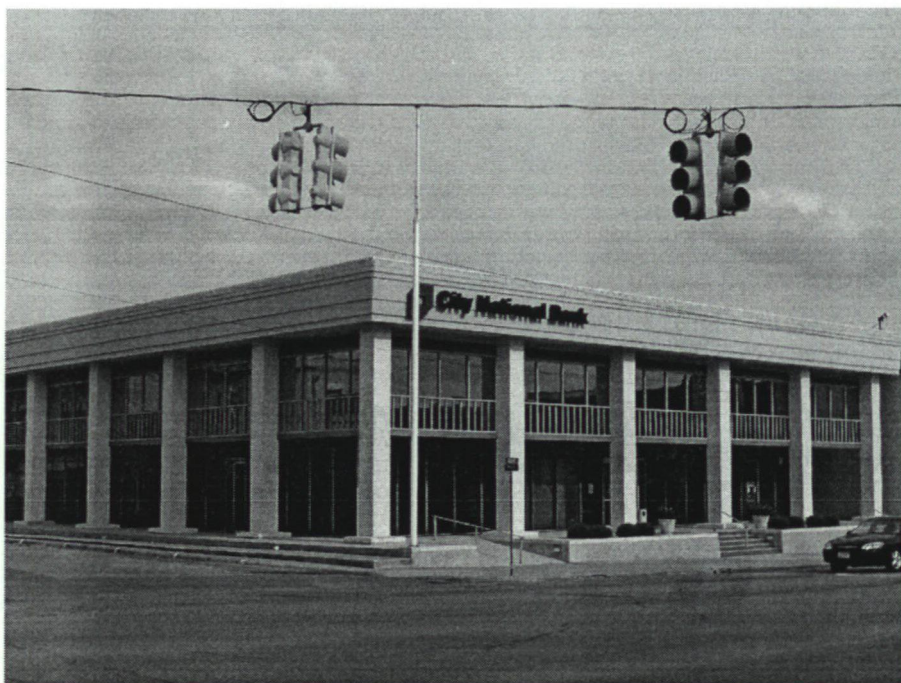
City National Bank (1965) 212 North Main Street Property #49 One-part commercial / enframed window wall Non-contributing Photo #16
