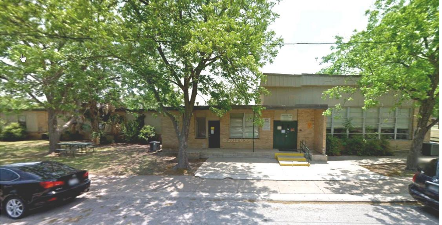
Figure 9 – “Band Hall” Annex Building – Site C
