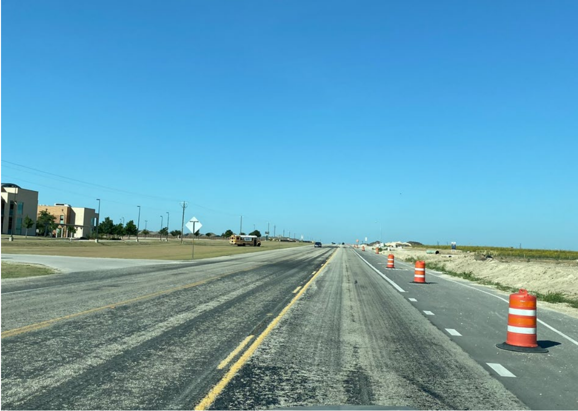
Photograph 3. FM 973, Looking South, at Taylor High School North Driveway
