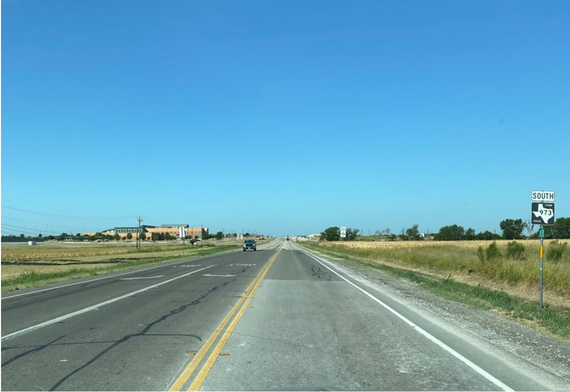
Photograph 2. FM 973, Looking South, South of US 79
