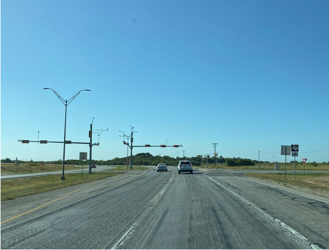
Photograph 1. US 79, Looking East, West of FM 973
