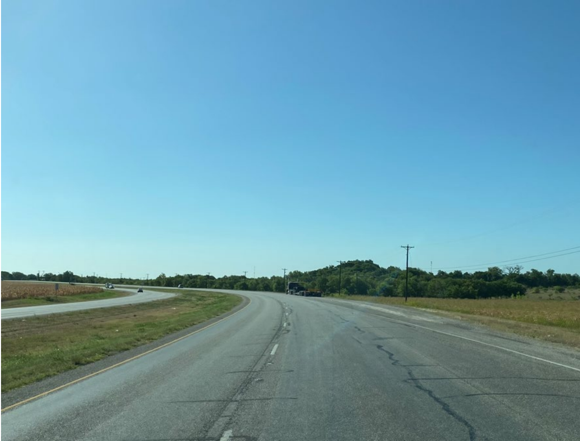
Photograph 5. US 79, Looking East, East of FM 973 Proposed site driveway (2A) to right.
