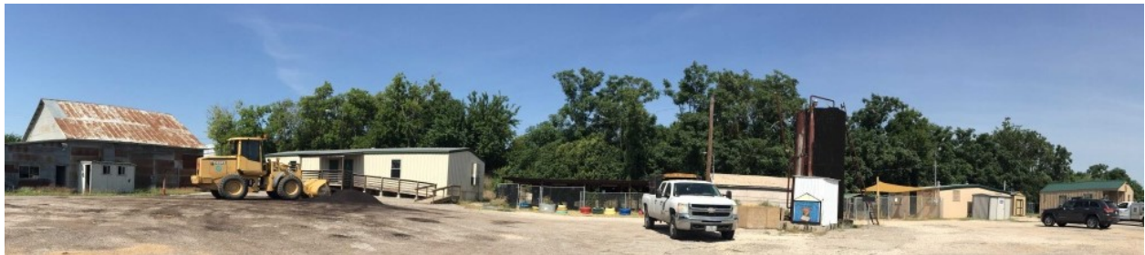
From left to right: Storage Barn, Portable Storage Building (from Taylor ISD), Outdoor Dog Kennels, and Laundry/Cat Room, Indoor Kennels, Food Storage Shed and Shelter Office.
