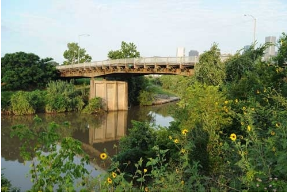
Hill Street Bridge, Houston
