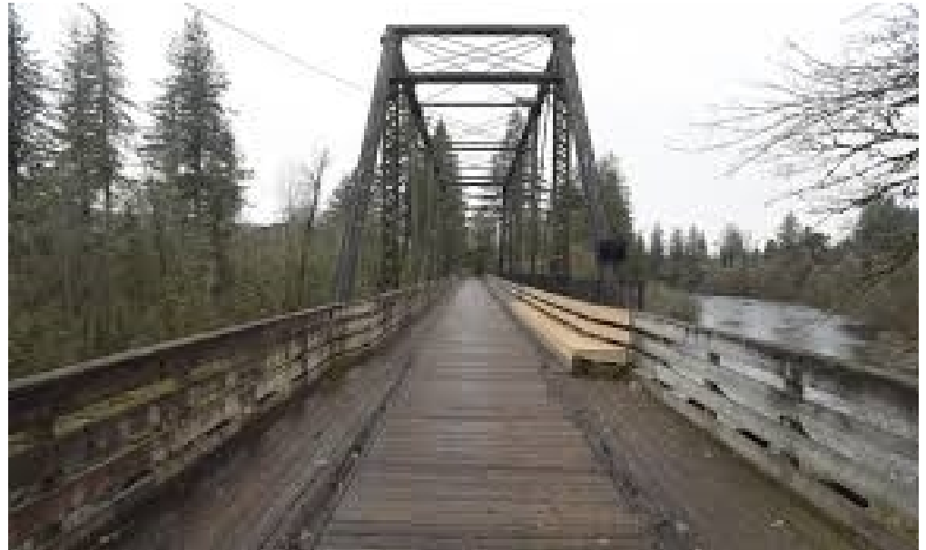
Mill City Bridge, Albany, OR
