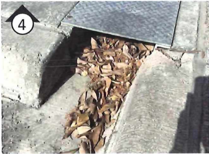
Keep drainage channels clear of debris.
