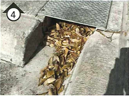
Keep drainage channels clear of debris.
