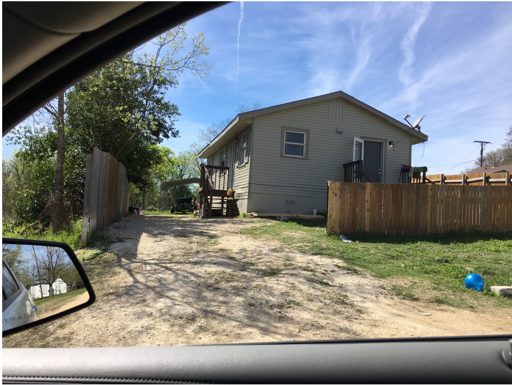
ATTACHMENT C - SITE PHOTO TAKEN 03-21-18
