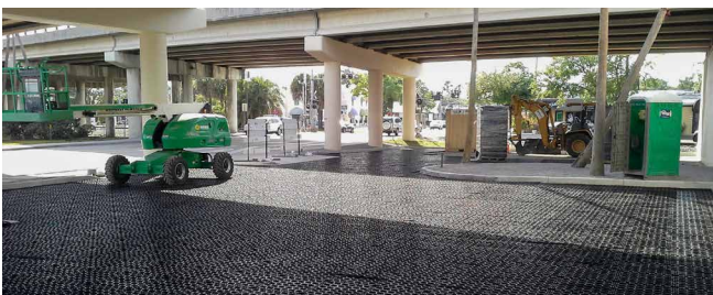
FLODOT Underpass Project
