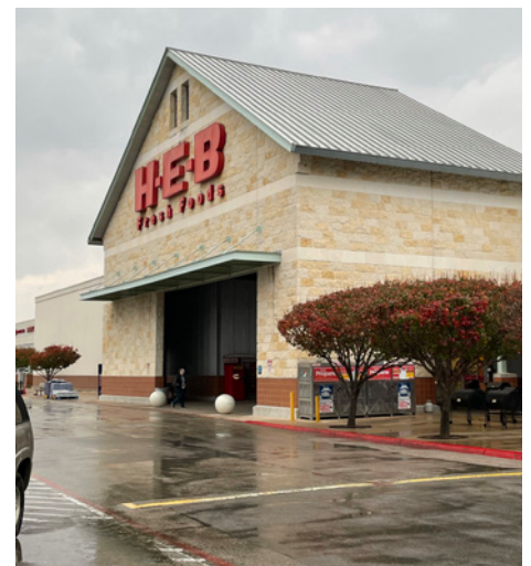
Retail centers drive vehicular trips Source: HDR
