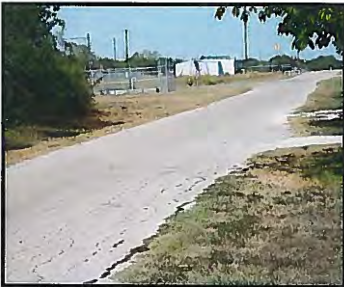
CDBG Wastewater Improvement Project Runge, Texas
