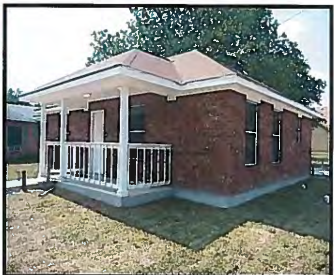
Home Reconstruction Project Taylor, Texas
