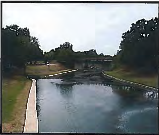
CDBG Riverbank Stabilization Project
