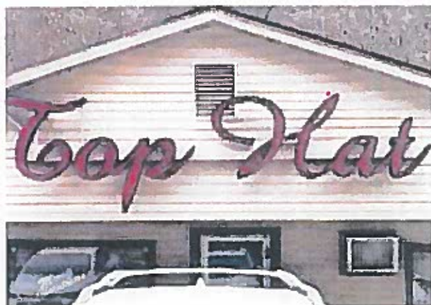
The internally-lit plastic sign is too large for this building's pediment.
