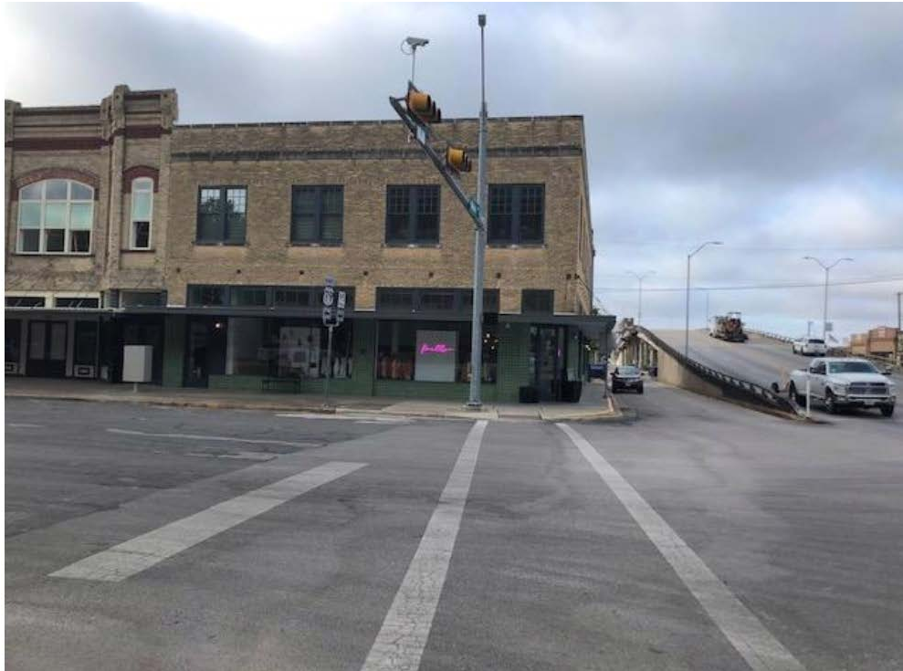
View from East Second Street
