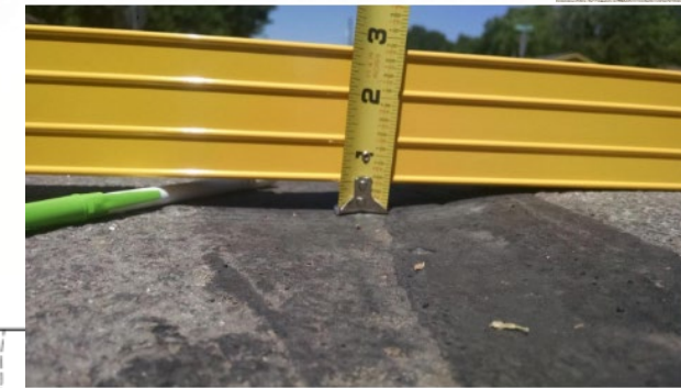
Figure 2: Displacement of 4th Street Pavement
