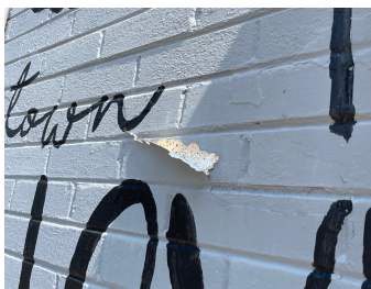
Scrape any areas of loose paint and spot prime as needed before painting
