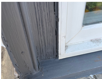
Repair with bondo
