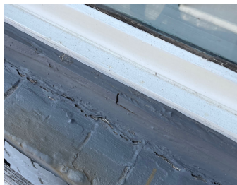
Repair with bondo
