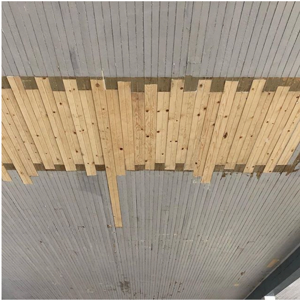
Ceilings repaired where necessary.
