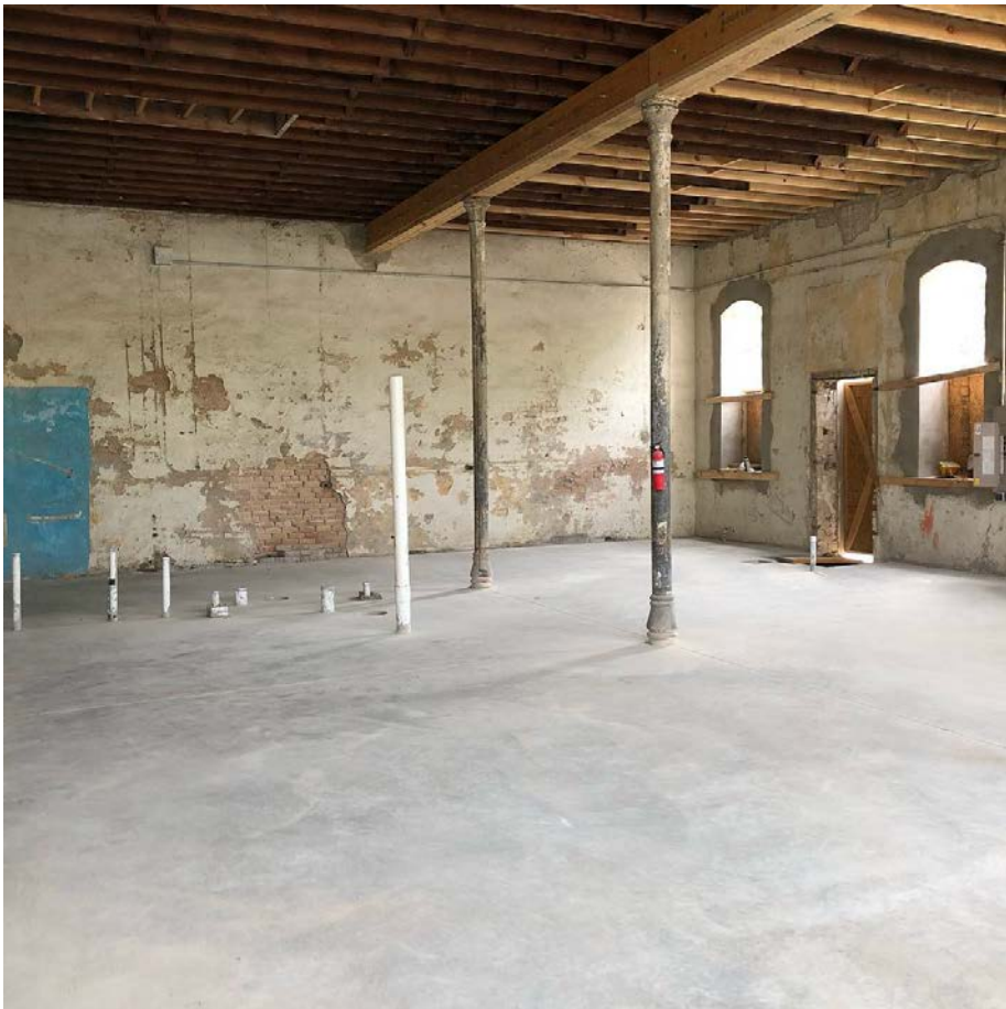
New concrete floors poured.
