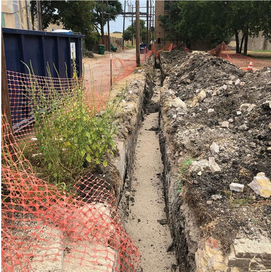
Water lines being installed.
