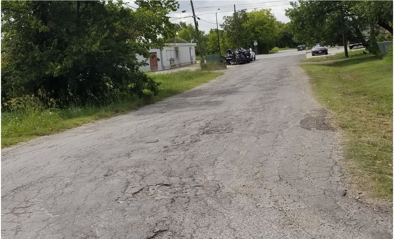
Poor condition pavement
