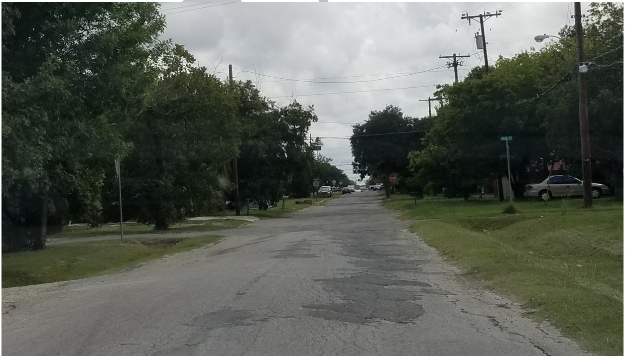
Poor condition pavement
