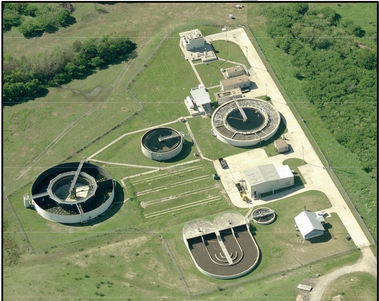
Figure 9-1. “Bird’s Eye” View of WWTP Property
