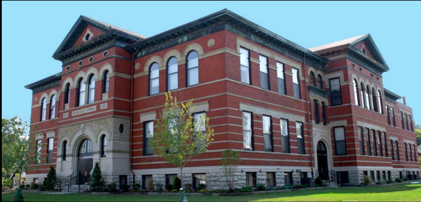
Academy Flats, Covington, KY , 26 units
