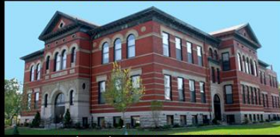
Academy Flats, Covington, KY , 26 units
