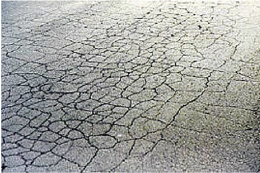
Alligator Cracking
