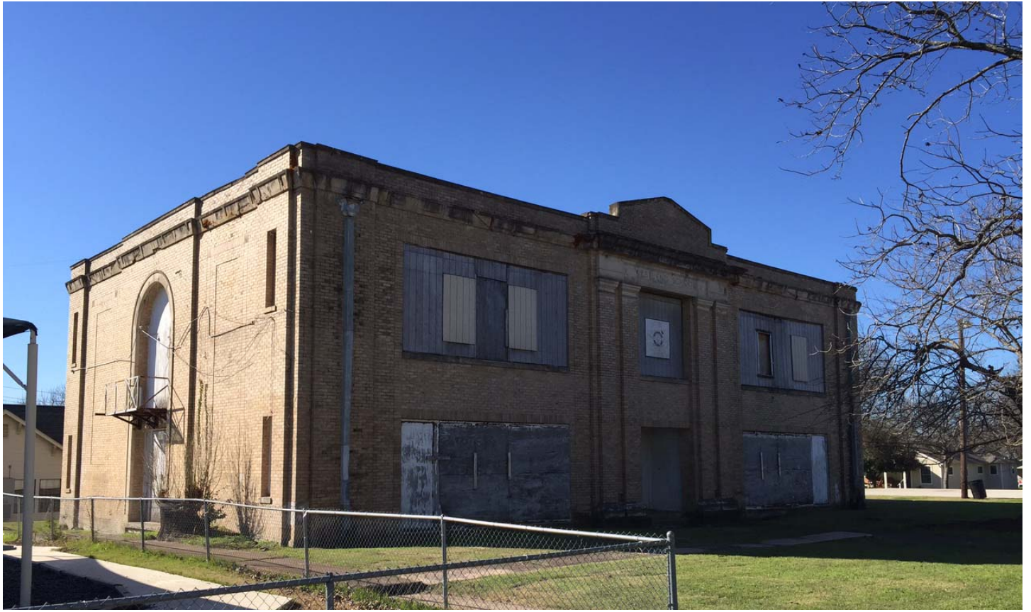
Figure 2 – West End School Building
