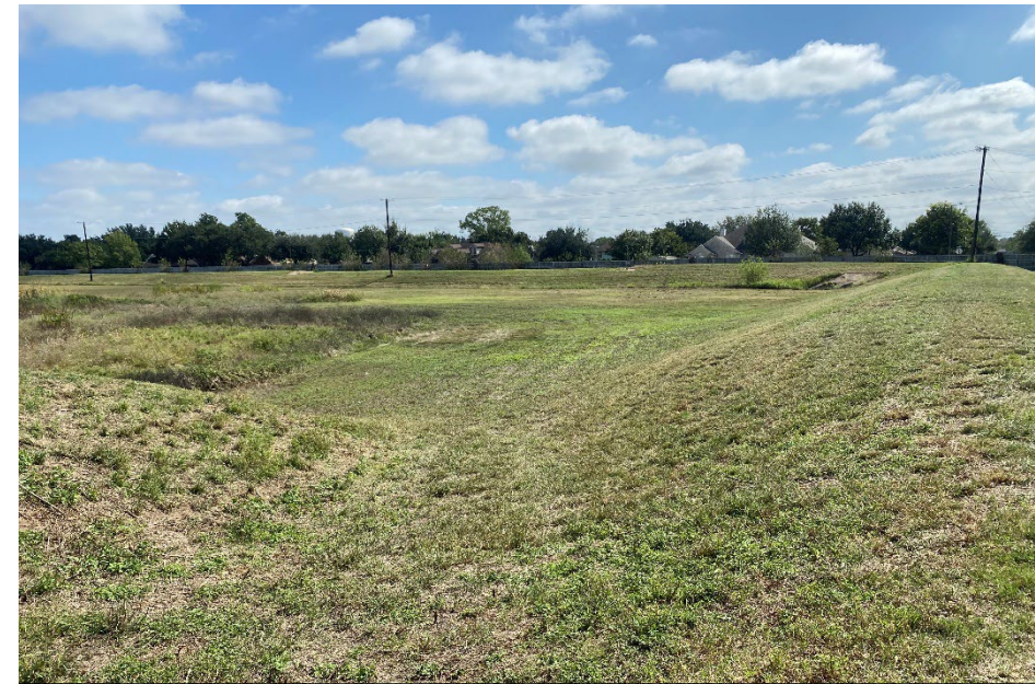
NW corner of pond looking south, low point in berm
