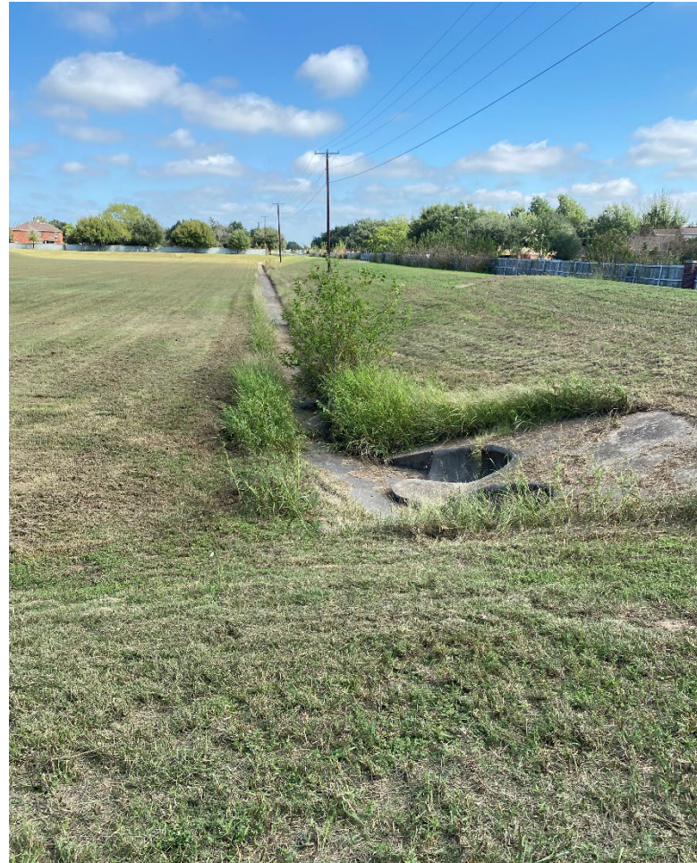
Pond concrete channel and outfall, looking east
