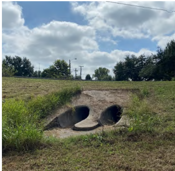
Figure 1: KBI Pond principal spillway: two 36-inch RCP
