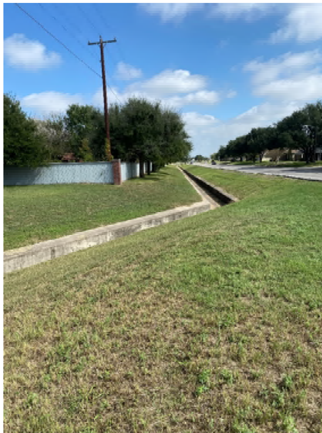
Figure 3: Concrete drainage channel entering pond, looking east
