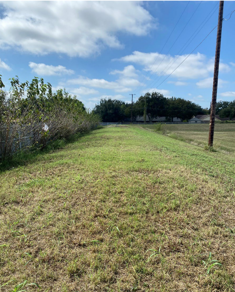
Pond emergency spillway, looking west
