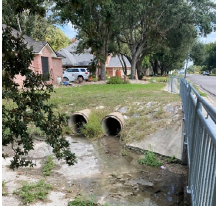
Figure 2: Outfall of pond principal spillway into neighborhood drainage channel (1310 T.H. Johnson Drive)
