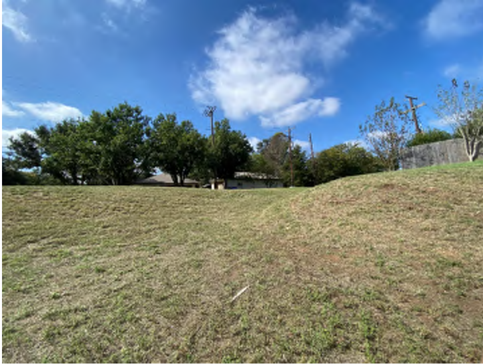
Figure 6: Saddle in northwest corner of the pond berm (elev. 595.89')
