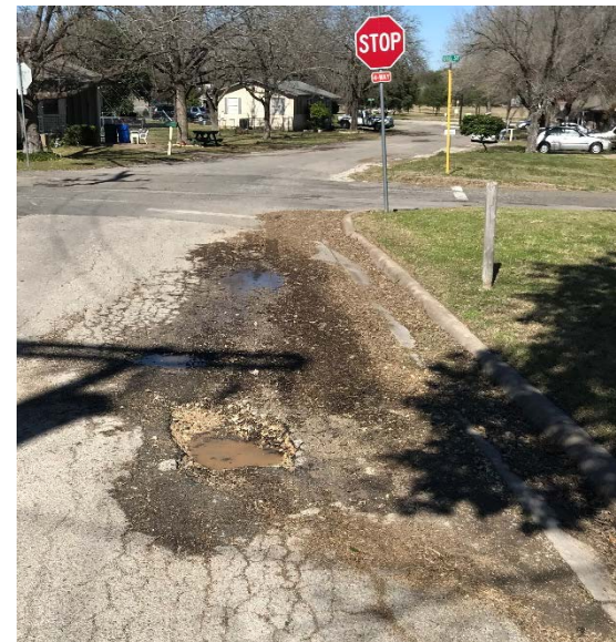
Pavement Surface Damage on N. Lynn Street (Above)
