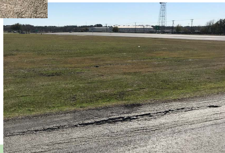
Pavement Surface Damage on N. Lynn Street (Above)
