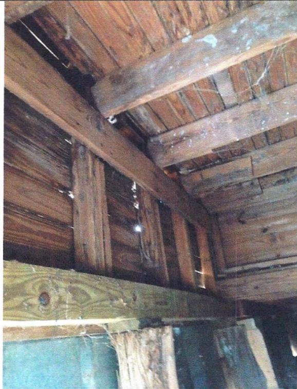
Underneath stage, northeast corner.
