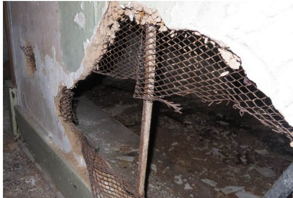
Figure 6: Typical smaller room and closet plaster wall with lath.
