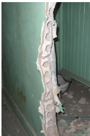
Figure 5: Typical hollow clay tile at corridor walls.
