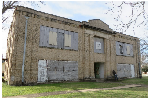
Figure 1 Front (north) wall of the West End School.
