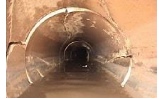
Infiltration (cracked pipe)
