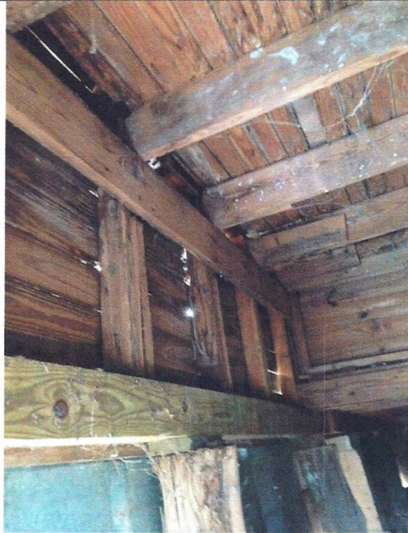
Underneath stage, northeast corner.
