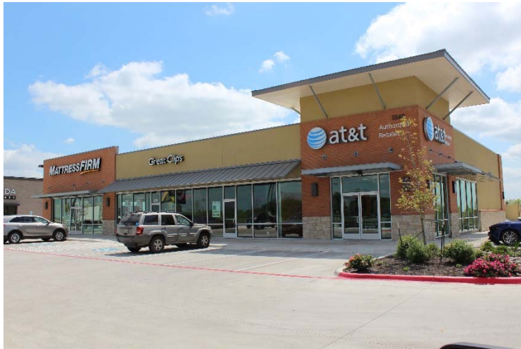
Unprotected Strip Center
