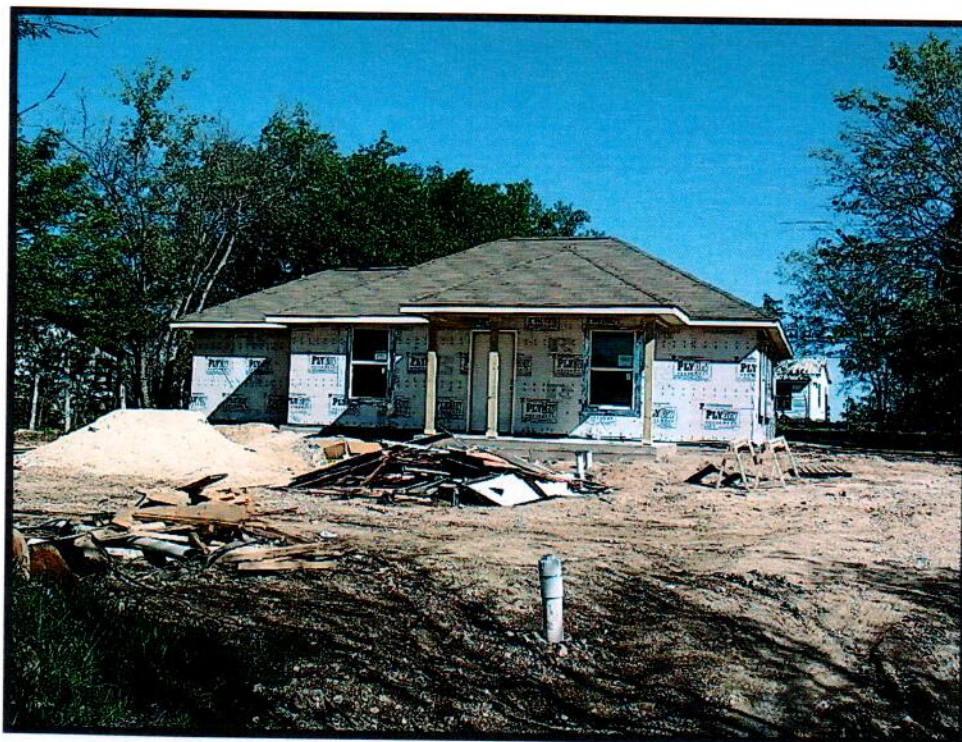
HOME HRA – Construction of a new home administered by LCMS
